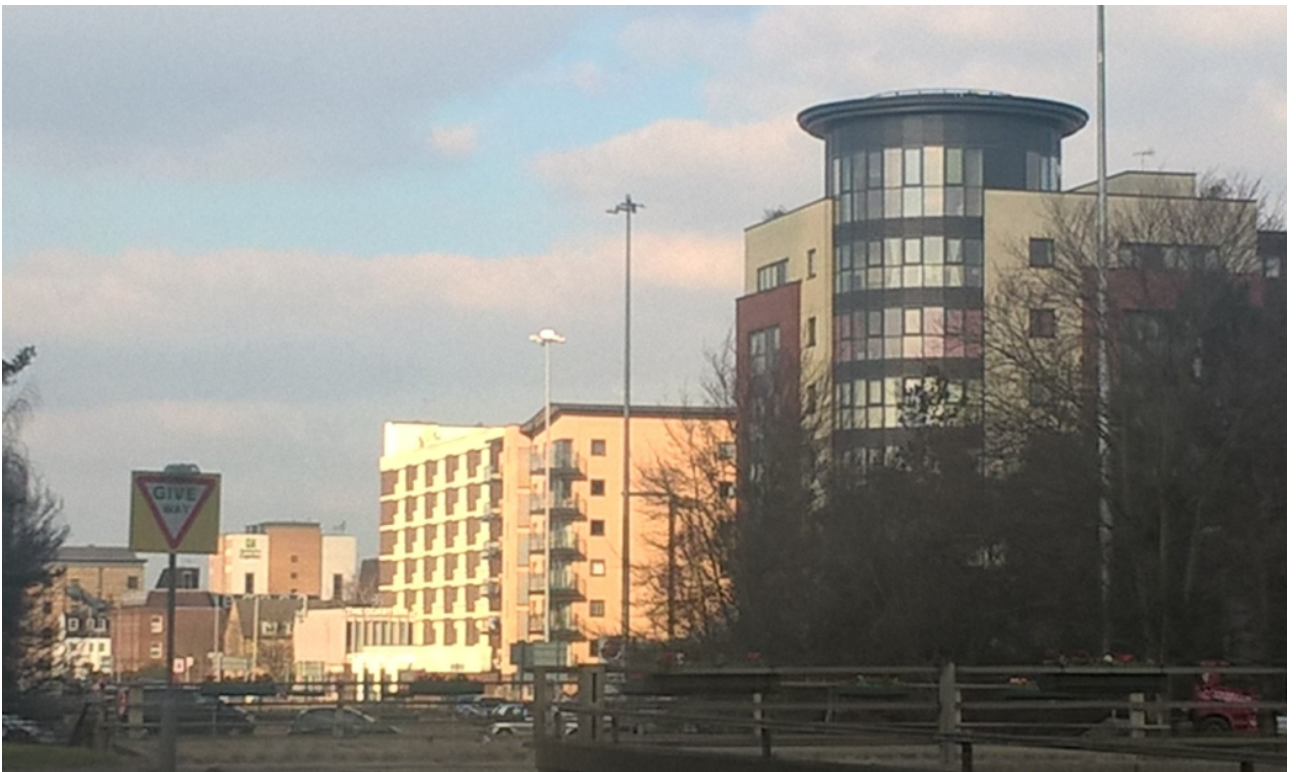
Fig. 2. View towards multi-storey buildings on eastern side of St. Albans Road.
